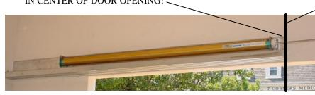
Above the left hand side of door opening install track w/ operator As shown in Figure B
